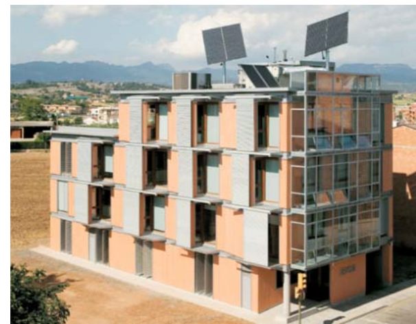
MANLLEU (SP) (Ecoedifici Lavola) / Office Small scale pilot Short term storage
